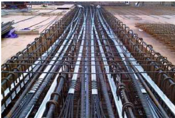
Figure 4. Using internal amplification «Internal Post-Tensioning»
