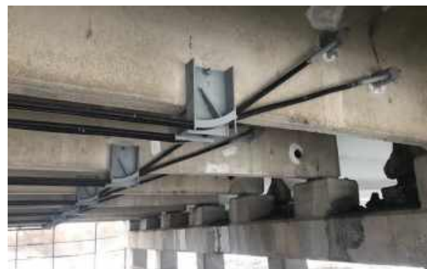
Figure 2. Use of external reinforcement "External Post-Tensioning"
