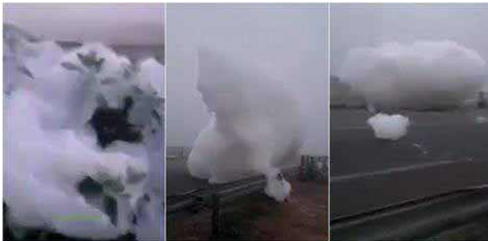
Fig.A-3.74 Excessive discharge of a foaming substance (for example, washing powder) into the sewer system causes foam to be released through cracks in sewer manholes (CC/GFDL)
